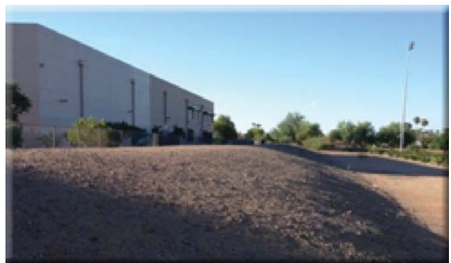
47th Avenue and Sweetwater berm - north dnd
