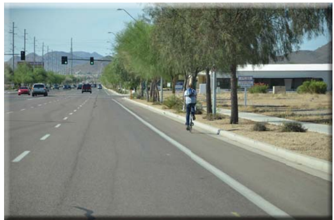
Bike lanes exist between SR-101 and Happy Valley Road (looking northbound)
