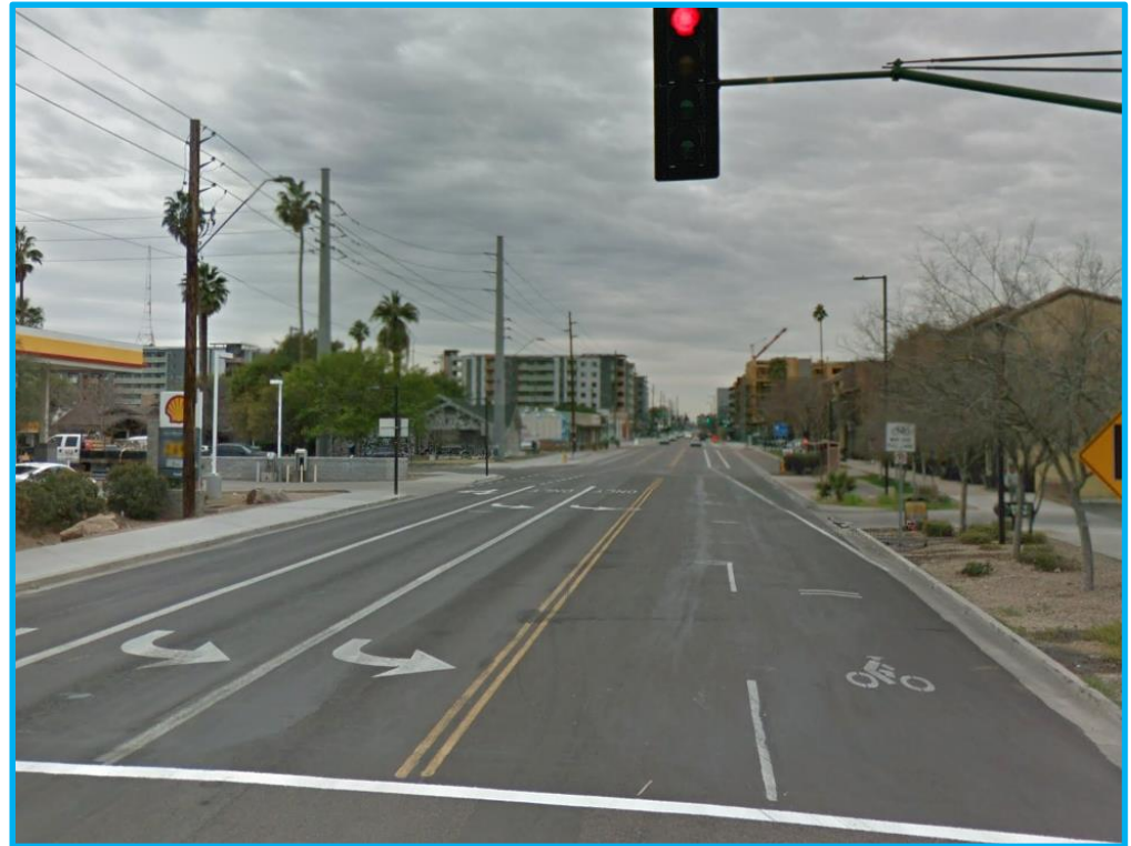
Shared-use bike lane markings on East Roosevelt Street west of 7th Street
